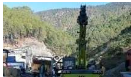
Hydra Crane for removal of Debris
