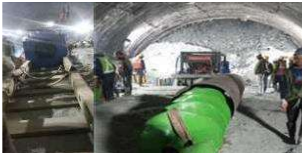
Connecting of Steel MS Pipe for inserting to initiate the safe evacuation.
