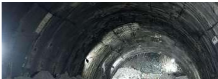
Iron Rib Protection work near the collapsed area for safety
