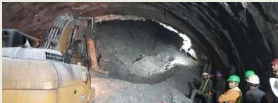
Section experienced the collapse and debris accumulated on the passage
