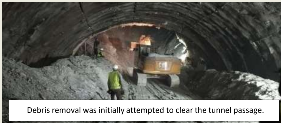
Section experienced the collapse and debris accumulated on the passage
