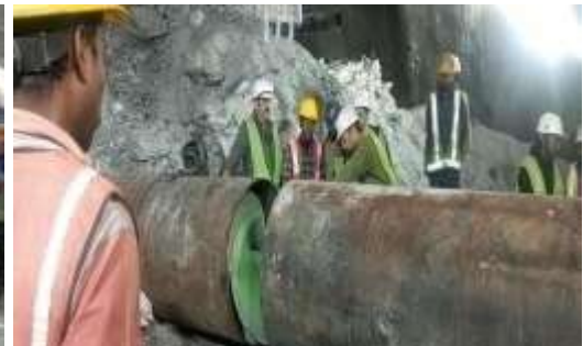
Connecting of Steel MS Pipe for inserting to initiate the safe evacuation.
