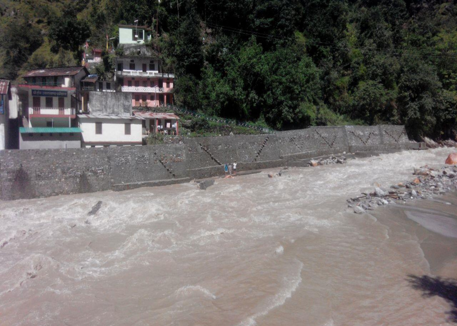
FPW AT KALIMATH IN KALIGANGA RIVER
