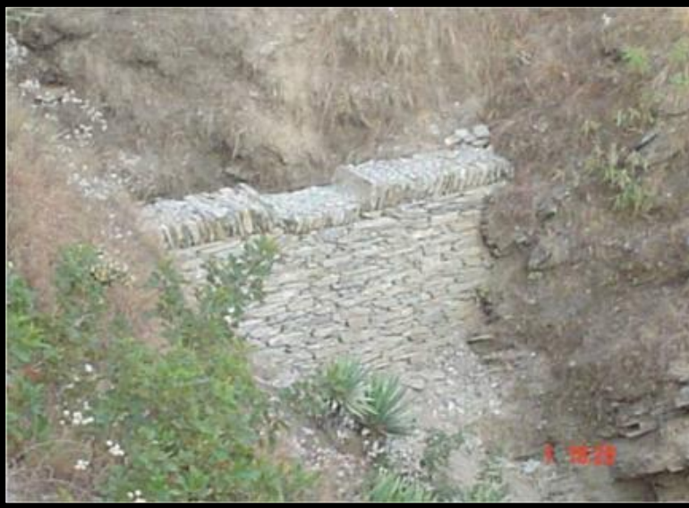
Dry Stone Check Dam
