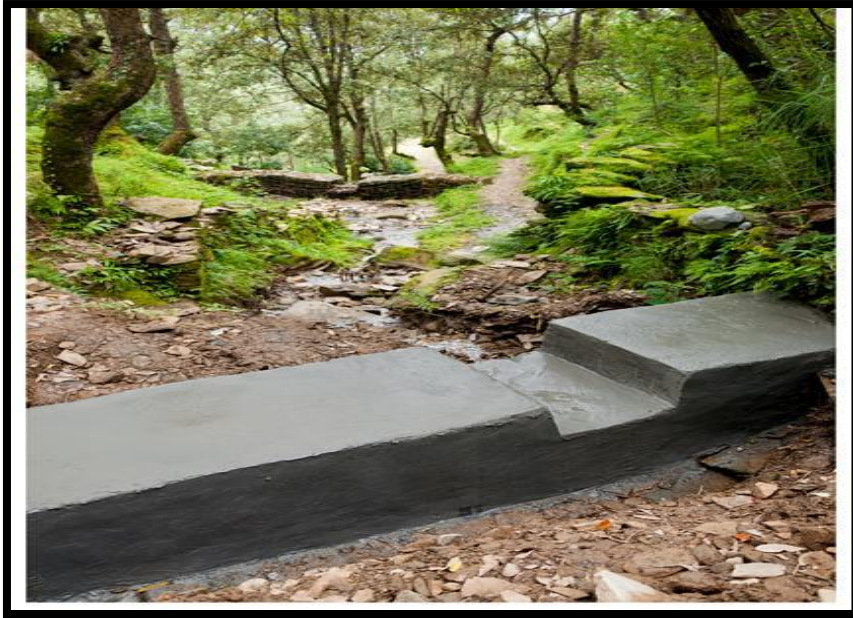
Sub Surface Check dam
