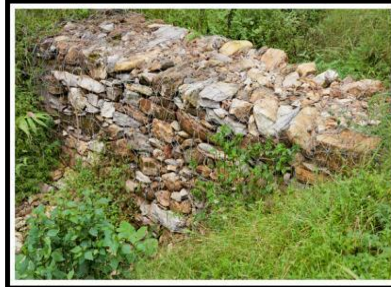
Gabion Check Dam
