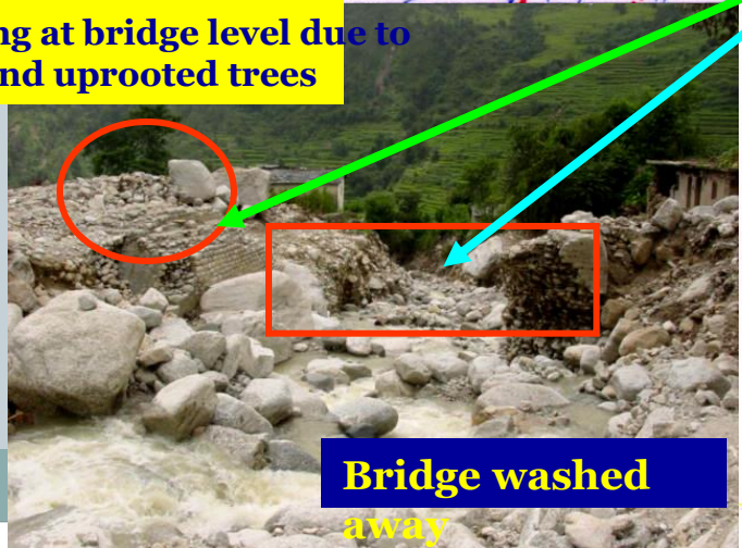
Changed flow of Nala Due to damming at bridge
