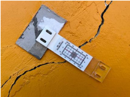
Installed crack meter on the wall
