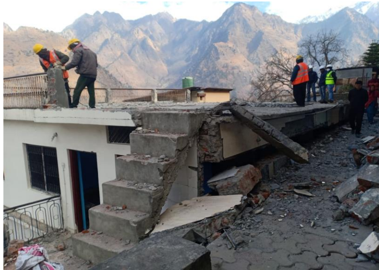
RCC building demolition
