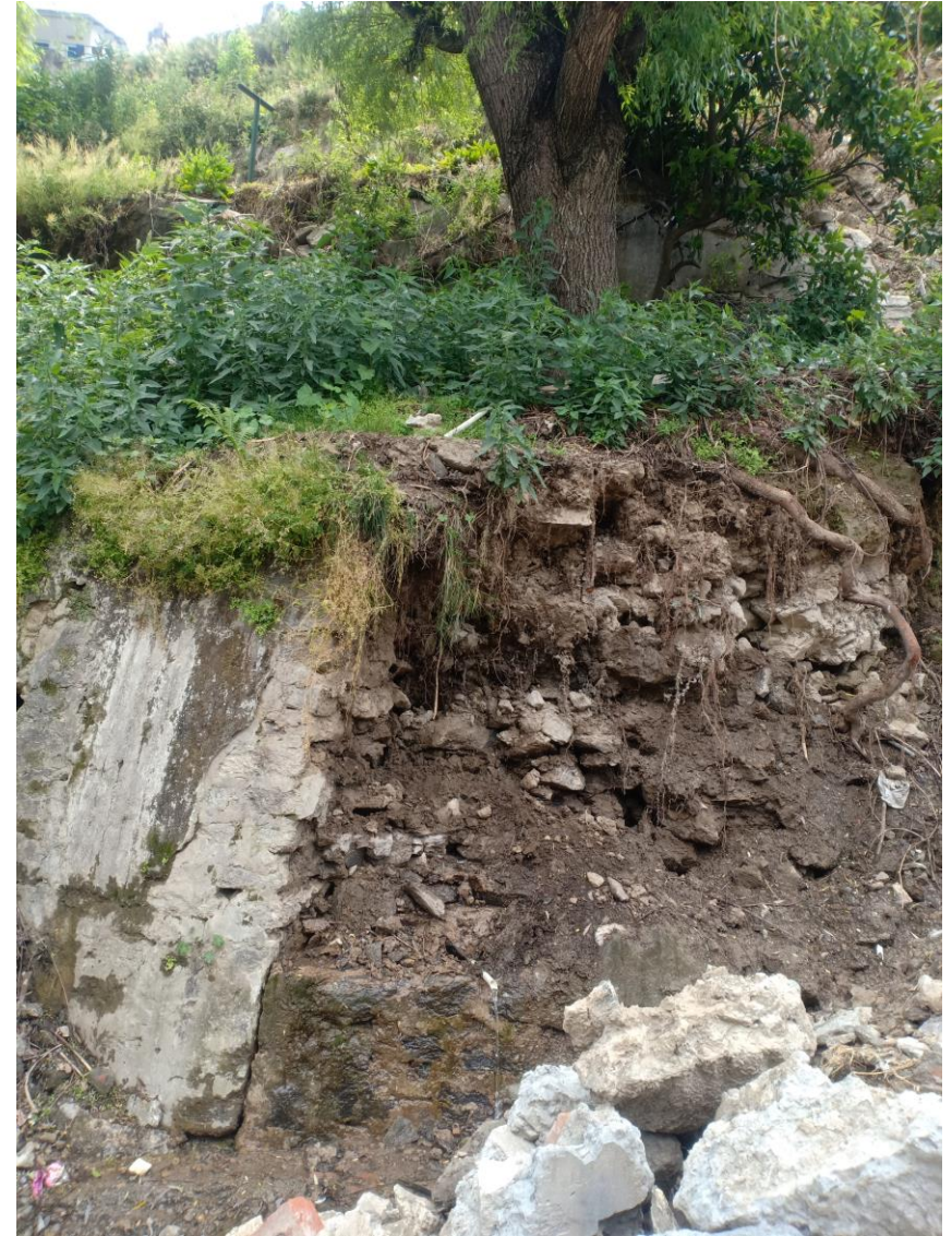
1 st Week of February 2023 , Fresh water observed in Jaypee Colony with a discharge of 5-10 lpm
