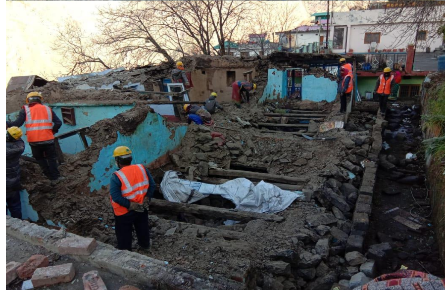
Stone-Mud mortar House under demolition
