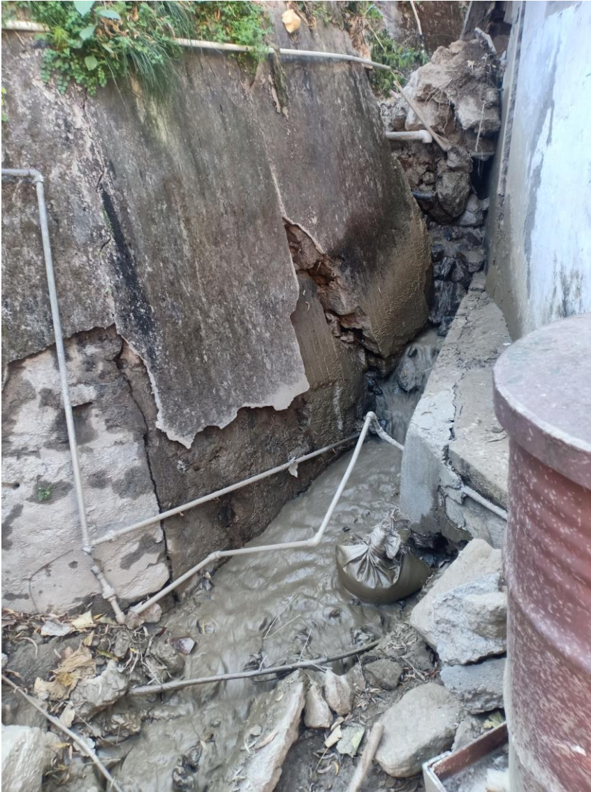
2nd January 2023 , Outburst of muddy water observed in Jaypee Colony with a discharge of 600 lpm
