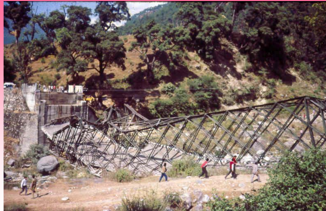
A Destroyed Bridge in Uttarkashi Earthquake,1991
