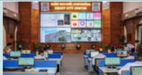
Central Control Room, Surat
