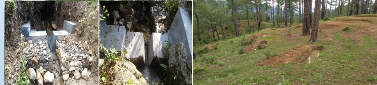
Figure: Kantali site and Contour trenches as a part of spring sanctuary in the catchment
