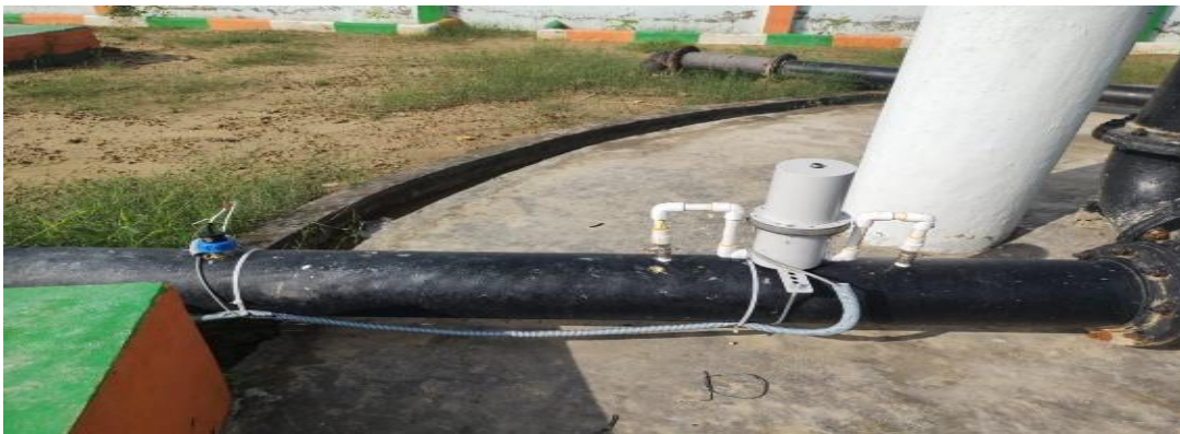
pH, TDS, Chlorine, Nitrate, Fluoride Sensor
