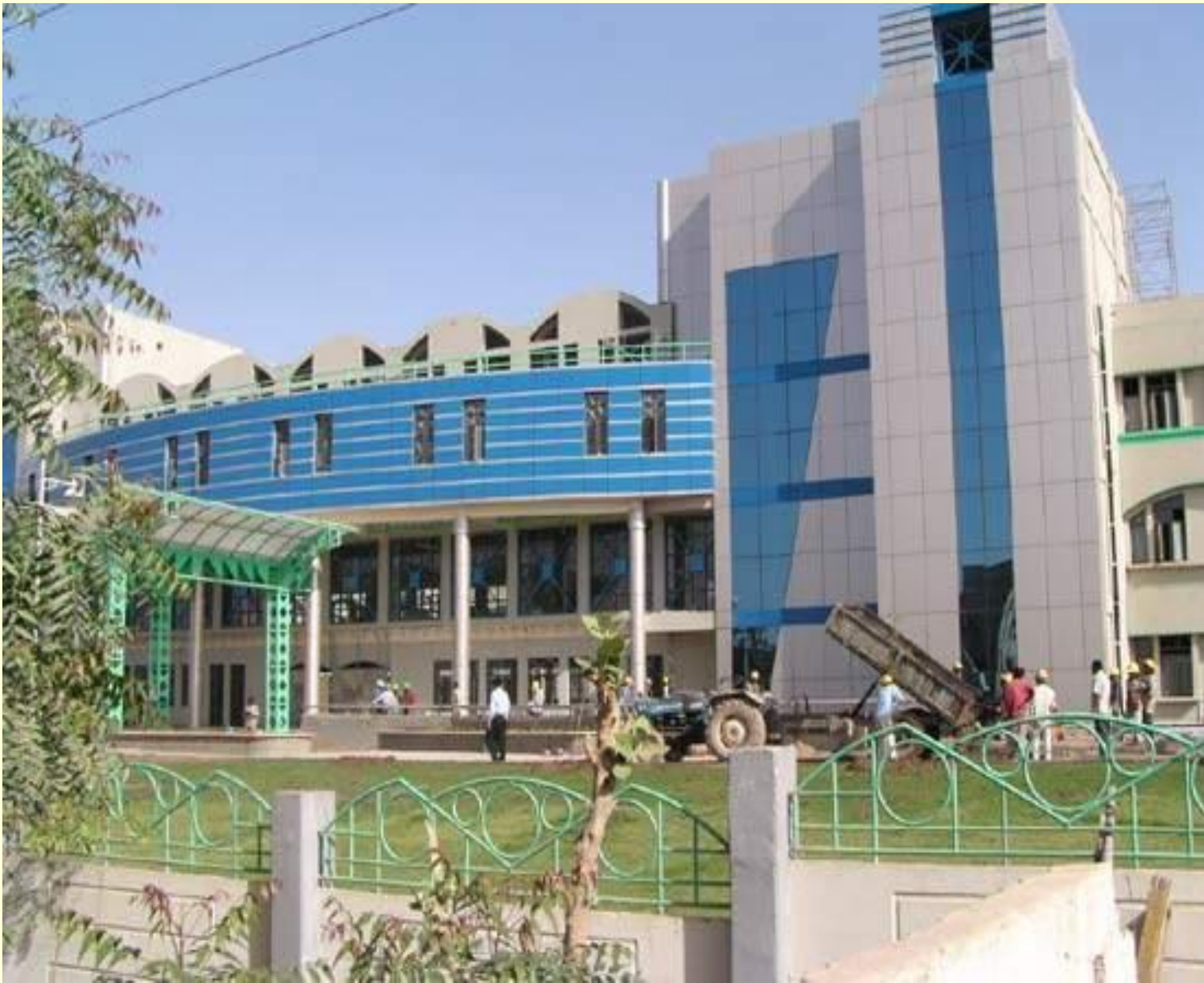
Bhuj Hospital is protected from earthquakes by lead-rubber base isolation system
